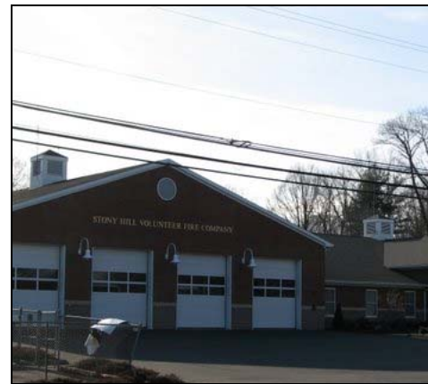
Stony Hill Fire Station
