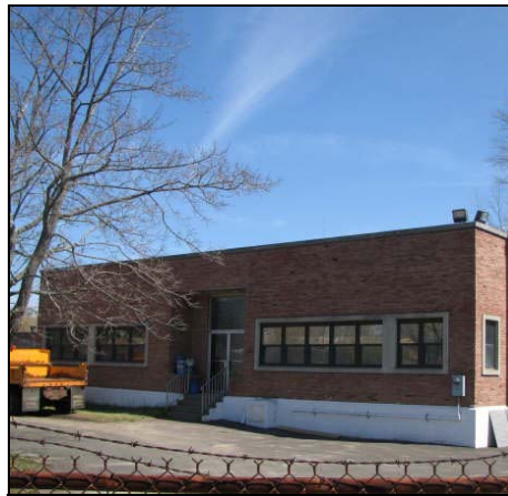
Sewer Pump Station
