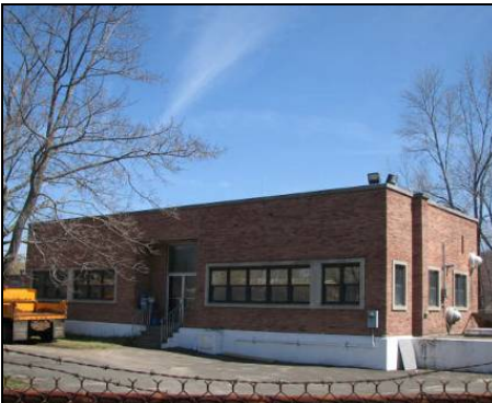
Sewer Pump Station
