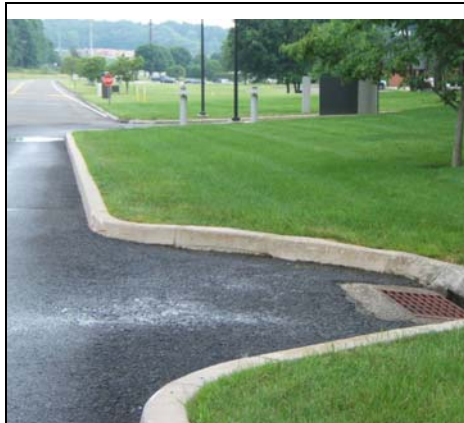
Road with Stormwater Management
